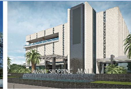
MARINA Shopping Mall-Uzbekistan
